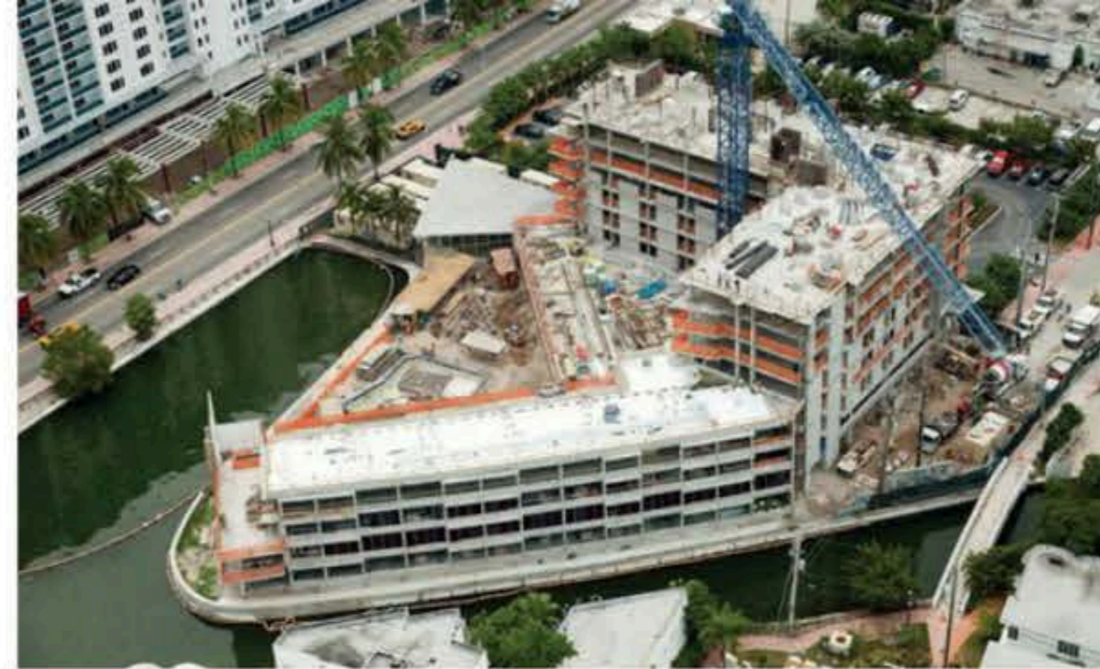
The Aloft South Beach Construction
